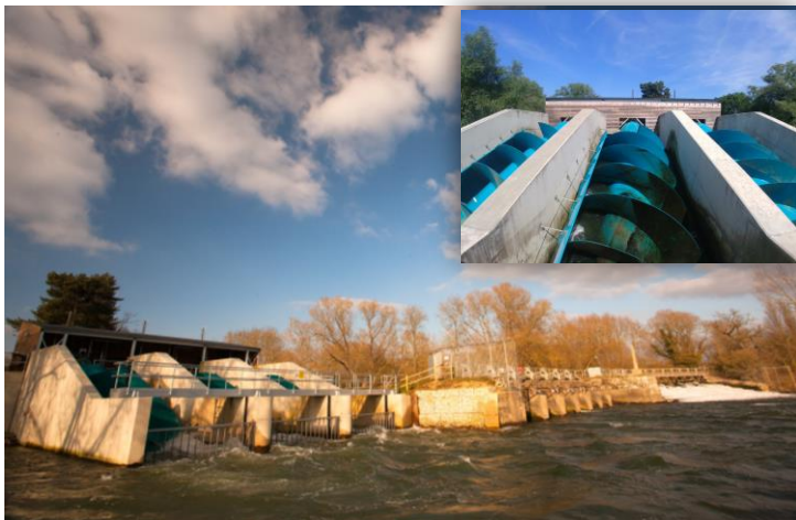
Sandford Hydro (Generation)
