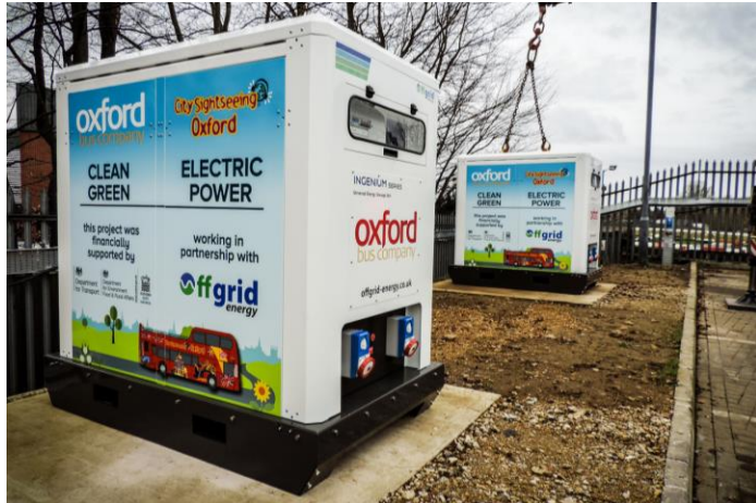
Oxford Bus Co. Batteries (Storage)
