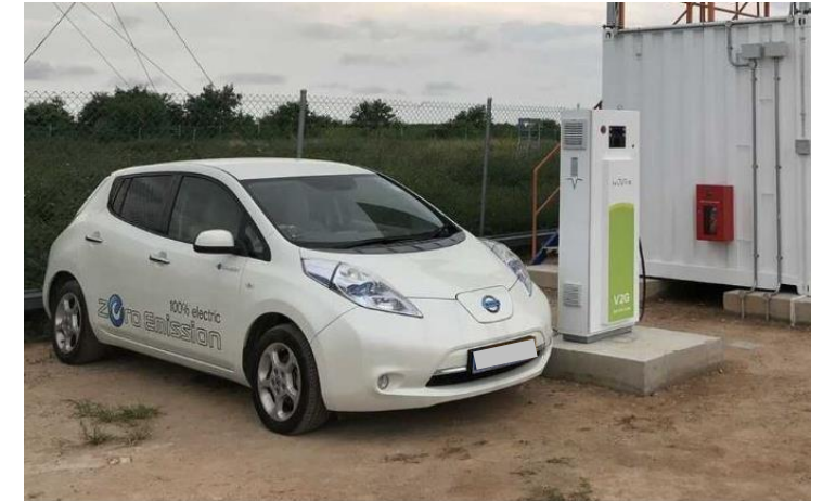
Nuvve 'Vehicle to Grid' chargers (Aggregation)
