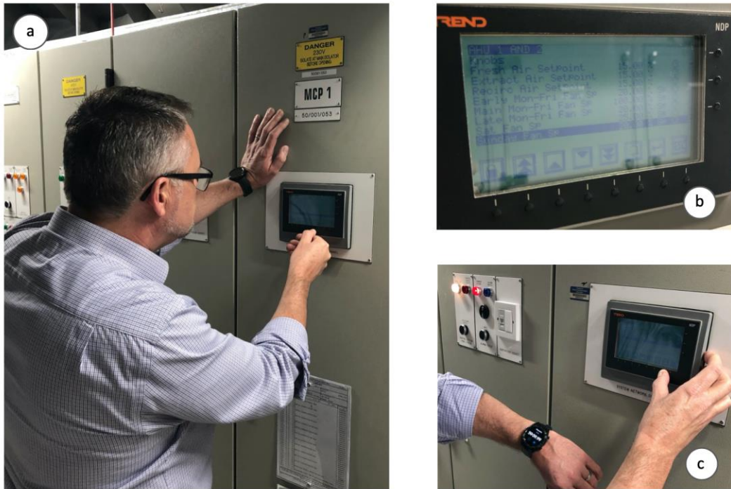
Figure 15: Engineer Martin Taylor (a) from the UoO Estates Management Team manually controlling the Trend BMS System (b) at the connection point for the MVS A3.1.2 trial which ran between 13:30-14:30 (one hour as shown in (c) ) on December 17 th , 2019.
