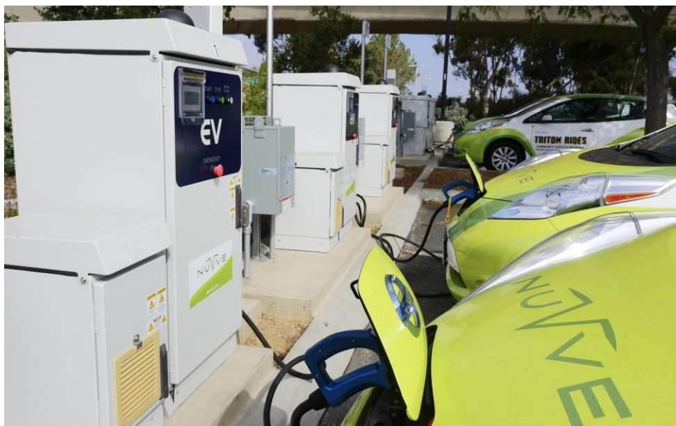
Figure 1: Nuvve vehicle to grid chargers deployed as part of the Invent project in San Diego, California USA. Source: Nuvve
