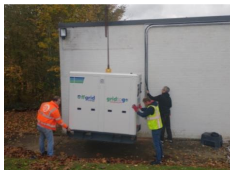
Figure 4: Rose Hill Battery being installed
