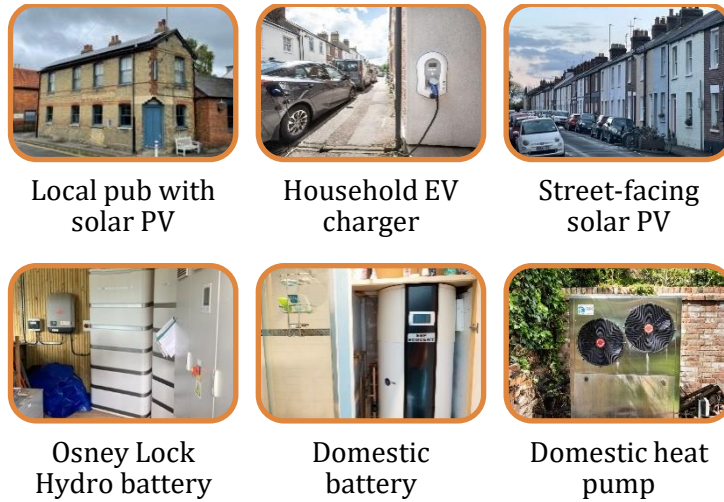
Figure 7: Osney Supercharge Smart Community Energy System elements (photo credits: Low Carbon Hub)
