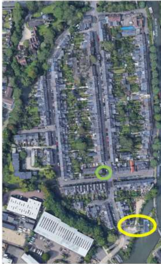
Figure 1. Satellite view of the Osney Island in Oxfordshire. The secondary substation is highlighted by the green circle, the Osney Lock Hydro in yellow circle (image from Google Earth).
